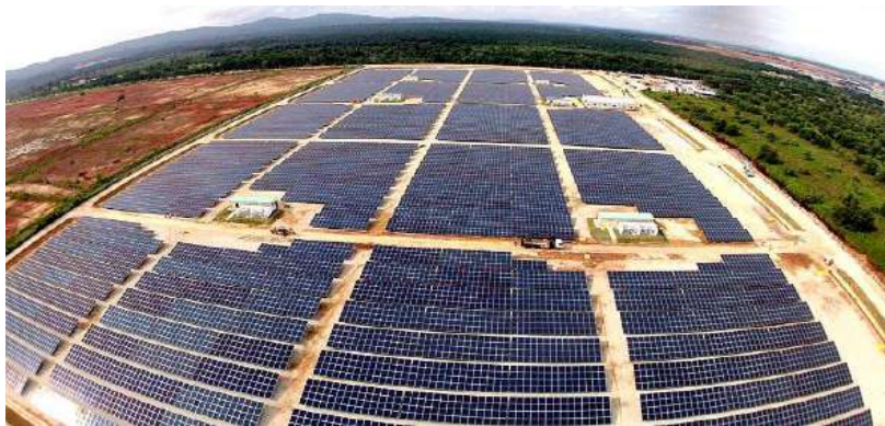
10 MW solar farm at Gebeng, Pahang, Malaysia
