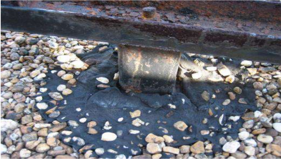
Corrosion
